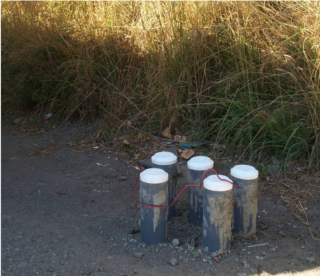
Figure 10. Verification cylinders at the job site.
